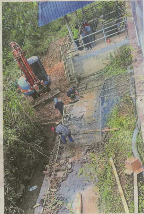
Plan B: Engineers and workers building an alternative water channel to the Kampung Bambang water intake point in Ranau.
